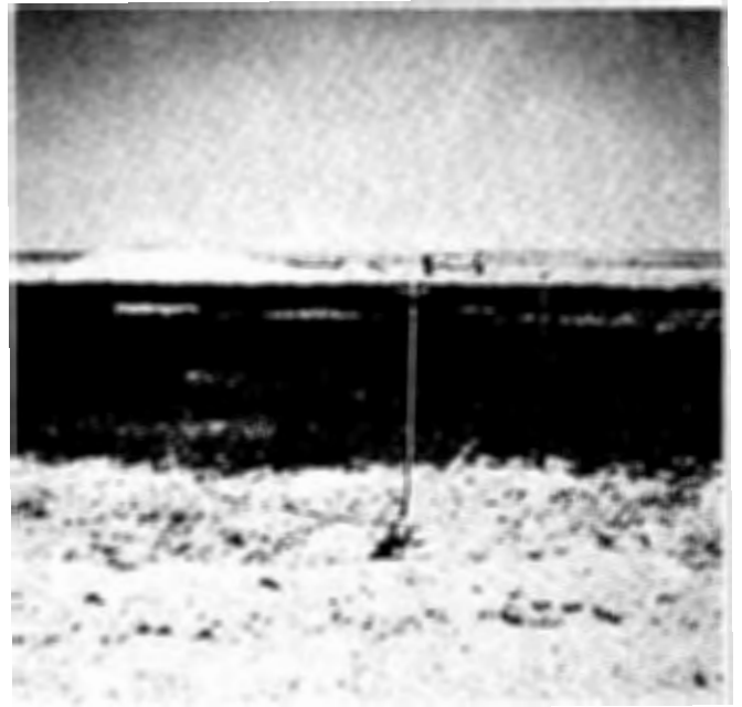
Demonstration plot of wheat and barley grown under sprinkler irrigation. Background, left, is a large concrete reservoir, protected by earth embankment, filled during the night by pumping from adjacent wells. Water is piped during the day to sprinkler heads.
