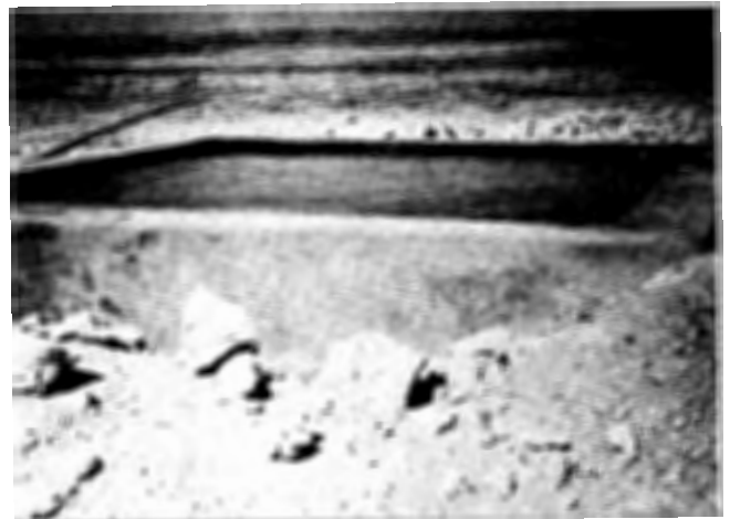
Small concrete reservoir with water piped in from new wells, to be drawn off as needed through a series of pipes to the sprinkler heads in the field beyond.
